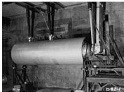
The Shrimp (code name Castle Bravo) device in its shot cab
